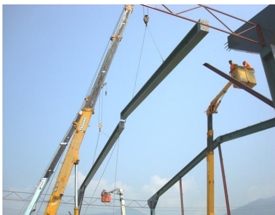
Figure 1 – Dura ® UB650 used in portal frame.
