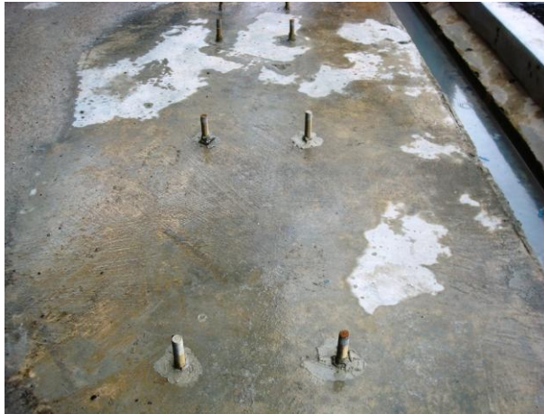
(a) Preparation of Drop-in Anchors on Floor.
