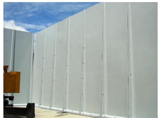
(f) Completed Wall.
