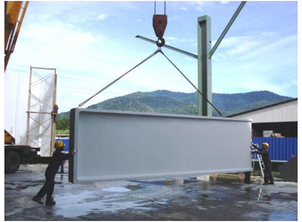
(b) Lifting of Wall WP70/20.
