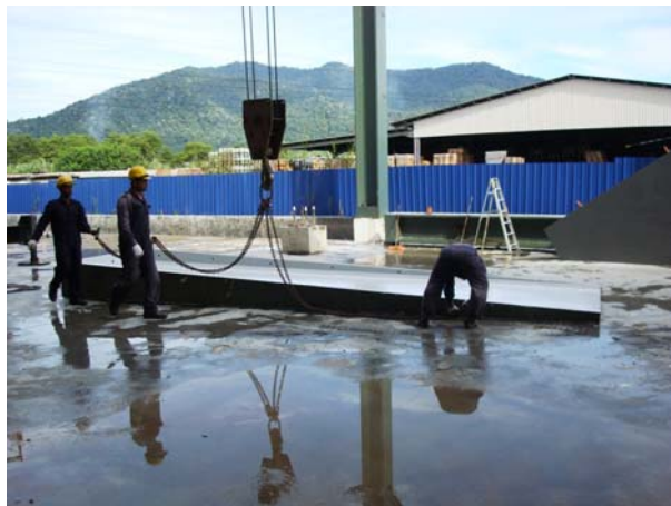
Step 3: Over-turning of wall
