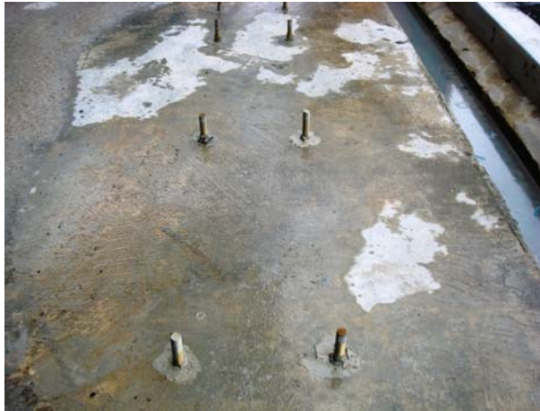
Step 1: Preparation of drop-in anchors on floors
