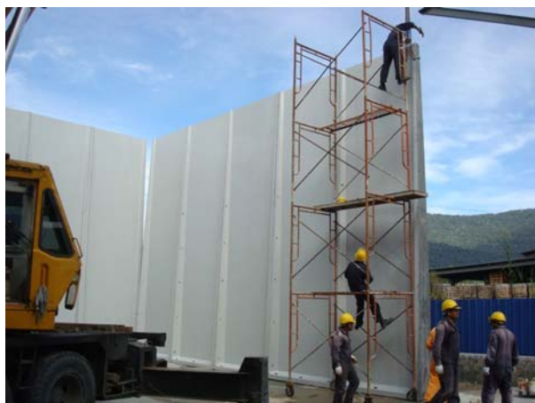
(e) Positioning and tightening to adjacent wall
