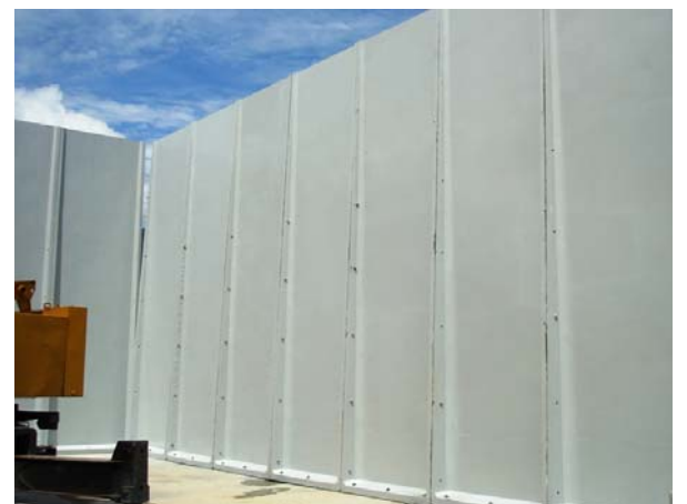
(f) Completed wall
