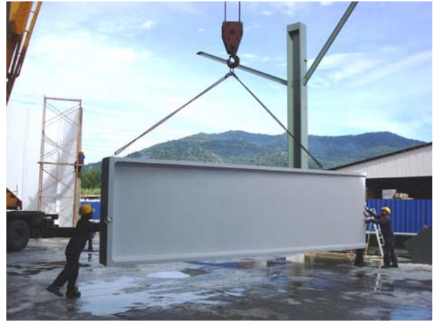
Step 2: Lifting of wall WP70/20
