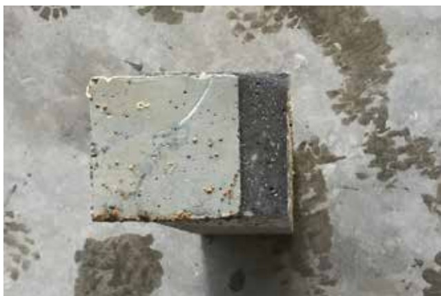
This 9 mm (0.35 in.) thick, saw-cut, eight-year-old sample from a high-salinity, long-term bath at Dura Technology in Malaysia shows corrosion on the surface only. Courtesy of J. P. Binard.
