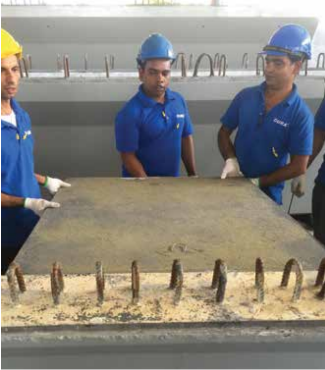
Dura Technology workers use waste ultra-high-performance concrete for a stay-in-place, noncomposite form for cast-in-place concrete deck placement. Courtesy of J. P. Binard.
