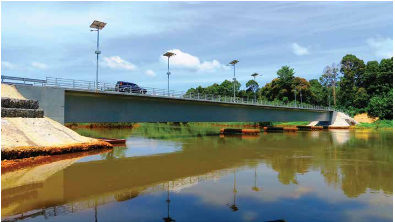
The segmental box-girder bridge at Batu 6 in Gerik Perak, Malaysia, is made with ultra-high-performance concrete and has a 328 ft (100 m) long span. Courtesy of Dura Technology.
