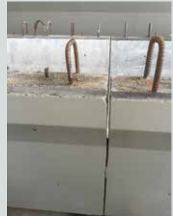
Rows of completed product are stored downline in tight increments to maximize the available space at the Dura Technology facility in Ipoh, Malaysia. Courtesy of J. P. Binard.
