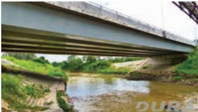
Figure 5: Rantau-Siliau Bridge. U-shaped UHPFRC girder with composite conventional strength concrete deck at different stages of construction: (a) and (b) during launching; (c) and (d) after completion.
