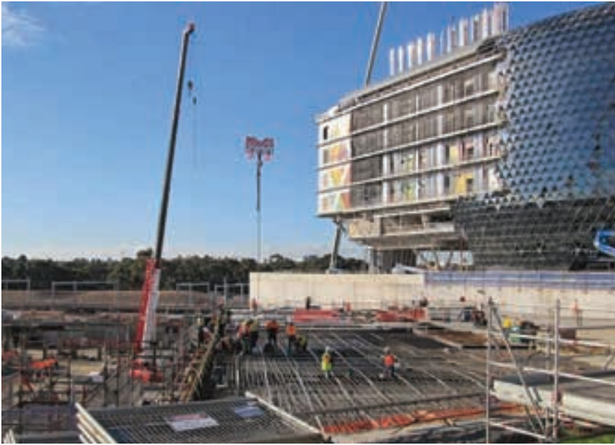
The Royal Adelaide Hospital under construction.
