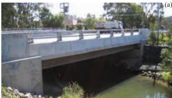
Figure 3: Shepherds Gully Bridge, NSW, Australia constructed in 2005: (a) 15 metre span 4 lane road traffic bridge (b) underside showing I-girders.
