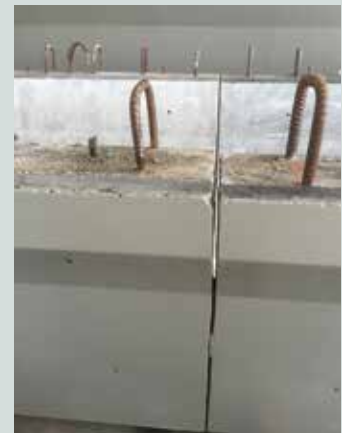
Rows of completed product are stored downline in tight increments to maximize the available space at the Dura Technology facility in Ipoh, Malaysia. Courtesy of J. P. Binard.
