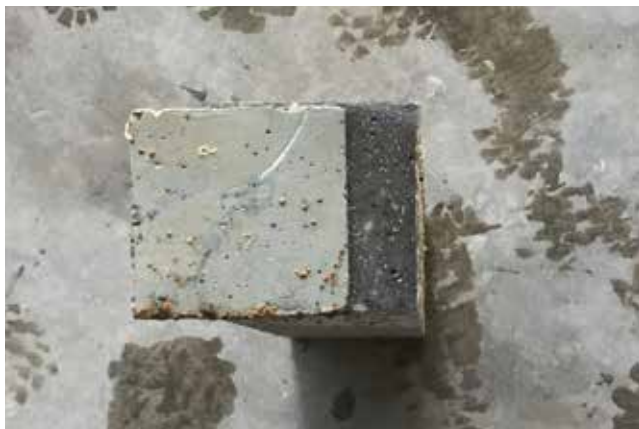
This 9 mm (0.35 in.) thick, saw-cut, eight-year-old sample from a high-salinity, long-term bath at Dura Technology in Malaysia shows corrosion on the surface only. Courtesy of J. P. Binard.
