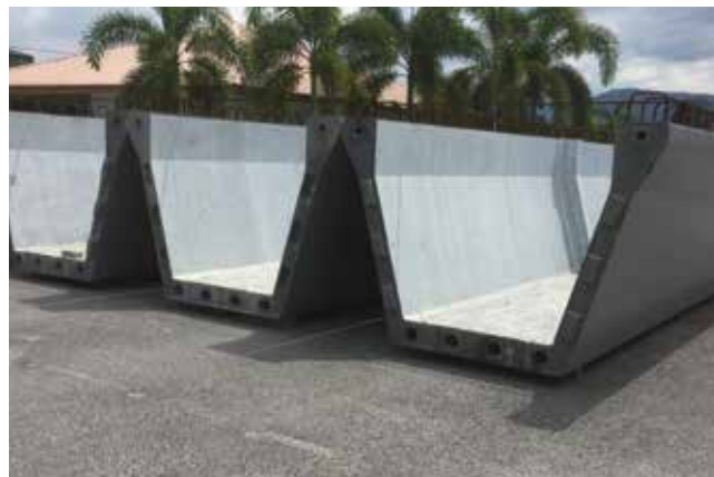
In storage at Dura Technology's facility in Malaysia, these U beams were produced with ultra-high-performance concrete and will be posttensioned in the field. Courtesy of J. P. Binard.
