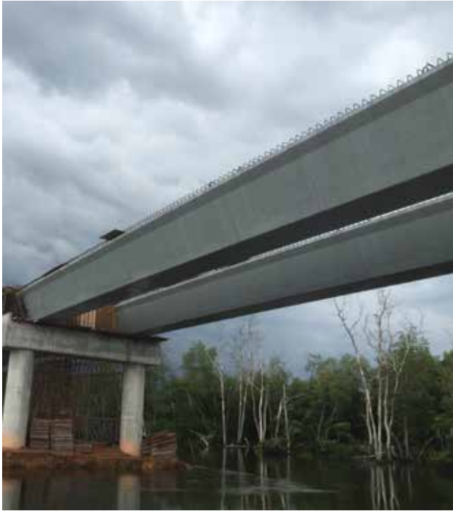
This 10-span bridge connecting Kampung Bahru and Kampung Teluk in Malaysia is shown under construction. Courtesy of J. P. Binard.
